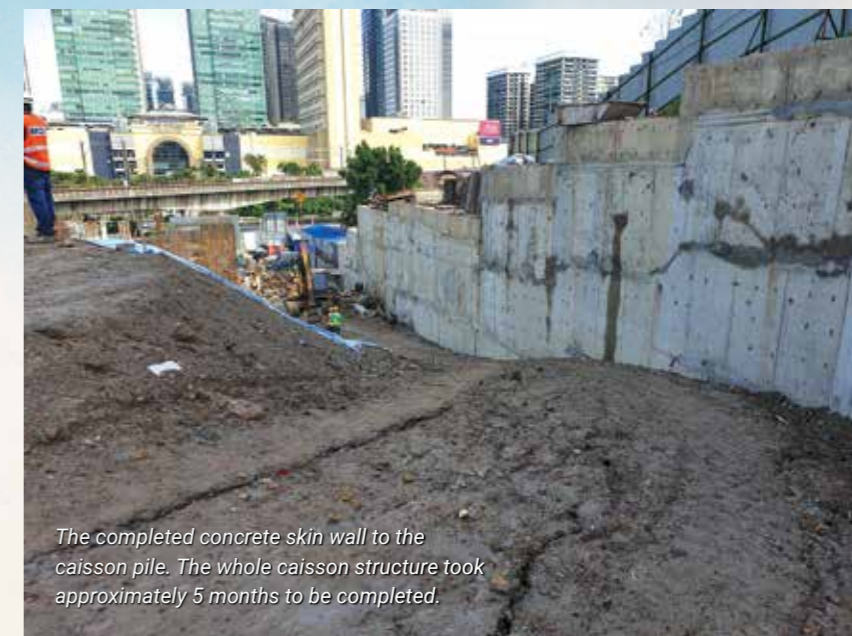
The completed caisson pile with capping beam.
